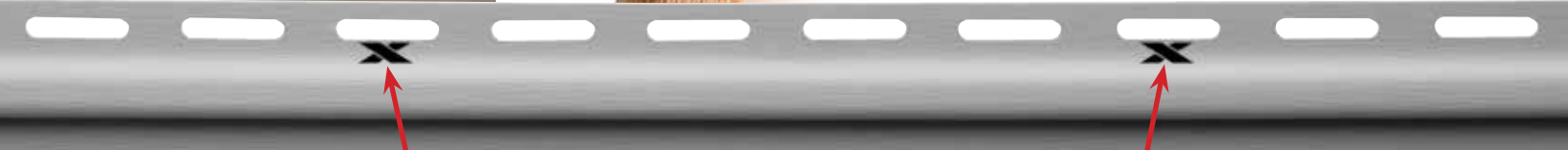
Unnecessary Nail Usage
